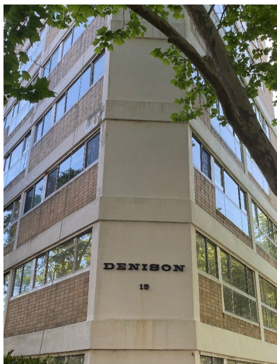
Figure 2 Denison on Wylde Street, Potts Point (1965), by Hugo Stossel & Associates, is a similar rectangular tower-form building with studio apartments off a central corridor. (Source: GML)
